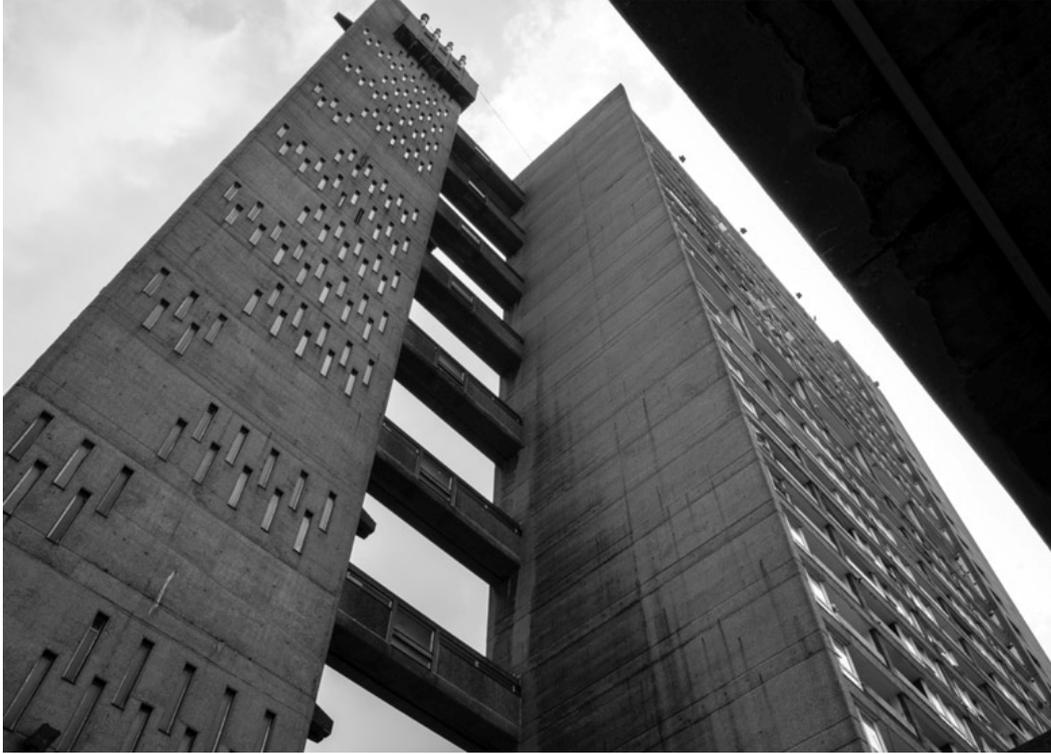
**Fig. 4** The Balfron Tower's detached elevator shaft from below.
